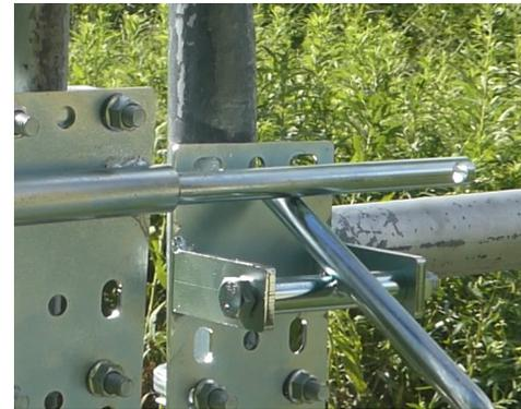
You need to adjust one of the brackets so that the bolt kicks the pendulum over then gets trapped behind it. As gates and posts tend to settle and sag, this adjustment is easy to make with a wrench or ratchet.
