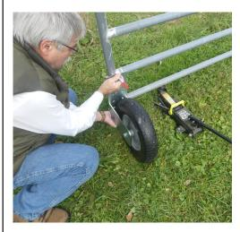
With the wheel mounted to the axel, put it up against the gate as shown, elevate the gate with the jack an additional ½", now mark where the top edge of the bracket should go.
