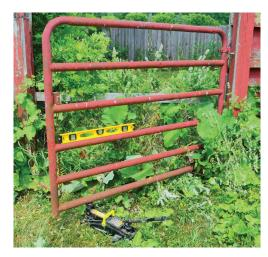
Level and Stabilize Gate - There are many ways to do this, but by far the easiest is to use a jack and a level as shown. This allows you to get the gate precisely where you want it and will also come in handy on the final installation step.
