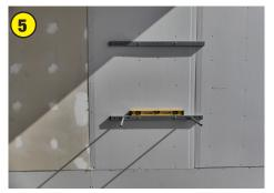
After you have mounted the upper rack, mount the lower rack 3-4' lower using exactly the same process with the level. Based on your preference and circumstances you may elect to put the rack that we're showing on the top in the lower position and vice versa.
