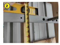
In this particular case the rack was 68" from the end of the boat and we are mounting this at 68" above the floor.
