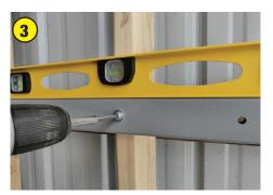
Secure one end of the rack with one screw, and then use a level to determine exactly what height the other screw should be. The process works extremely well and negates the necessity of measuring and the racks always come out level.
