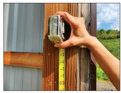
Measure the height at which you want to mount your lower lateral. After the lower lateral is mounted mount the upper lateral.
