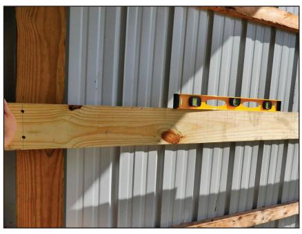
Use one bolt to loosely mount one end of your lateral. Using a level, level the lateral and then use a lag bolt to mount the other end. Screw in the lag bolts. Before screwing in the lag bolts, it would be a good idea to drill pilot holes half the diameter of the lag bolt.
