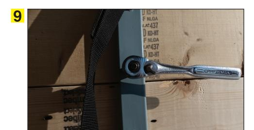
Secure the hooks to the laterals. Make sure you use at least 3 screws to mount each hook. Anything less may not be sufficient to properly support the weight of your boat.
