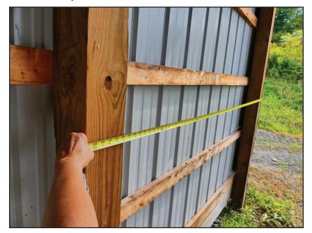
The first step is to measure the distance across the studs/uprights. This will assist you in selecting lumber of the appropriate length. In this case, our verticals are 16" apart and a standard 8' 2 x 6 works out to be a perfect solution.
