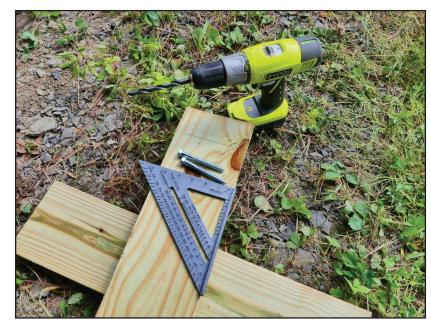
Once you have measured the location where you want to put your lower lateral lag bolts, mark it on your lateral and then drill through holes the diameter of the lags, as this will make it easy to screw them in, in addition to preventing splitting. For this particular project we have chosen to use  $\frac{3}{8}$ " x 3 ½" lag bolts and a  $\frac{3}{8}$ " drill. These would need to be purchased separately. Page 4
