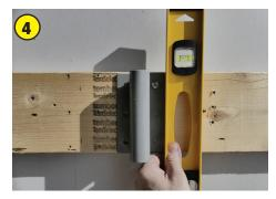
Use 6 screws to secure each hinge section to the 2''x 6" and then install the hook. Use a level to set the hinge vertical.
