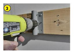
At the desired location put one of the hinges against the 2''x 6'', mark the locations of the holes, and then drill  $\frac{1}{8}''$  diameter pilot holes.
