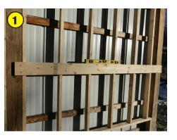
Typical wall studs are 16'' on center. Mount a 2''x 6'' across the studs and securely screw is to at least 3, preferably 4 of them, making sure that the 2''x 6'' is level. On drywall use a stud finder.
