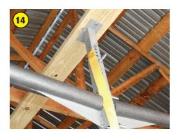
Have a 100mm M12 bolt in hand, and then slide the arm and extension assembly over the pedestal base that has been mounted to the mounting board and insert the bolt through the holes at the height that you determine to be best. The bolt should run front to back so that it doesn't contact the boat. Now tighten the nut. Repeat the same for the other bracket.
