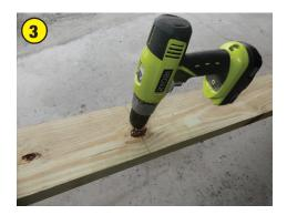
Pre-drill at least 3 holes at the rafter locations. A 3/16" diameter drill would be appropriate in most cases.
