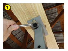
Tighten the lag bolts to secure the pedestal base to the mounting board. A ratchet will probably do the job easiest.
