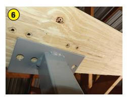
Measure the length of your boat and determine the spacing for mounting the brackets. Typically this would be 5-6'. Then put the pedestal portion of your bracket against the mounting board, mark the location for the lag bolt holes, and drill ¼" through pilot holes.
