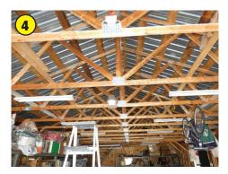
Use at least 3-4 #8 x 3" screws to secure the 2 x 6 or 2 x 8 at each intersection.
