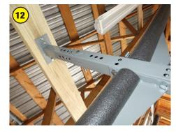
Have a 100mm M12 bolt in hand, and then slide the arm and extension assembly over the pedestal base that has been mounted to the mounting board and insert the bolt through the holes at the height that you determine to be best. The bolt should run front to back so that it doesn't contact the boat. Now tighten the nut. Repeat the same for the other bracket.
