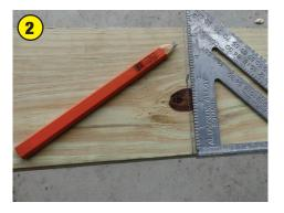
Measure the distances between the rafters and mark the center of each intersection accordingly on your 2x6 or 2x8.
