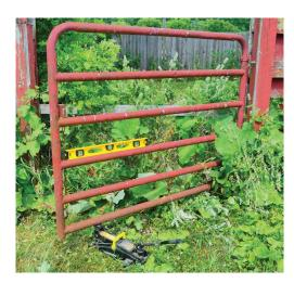
Level and Stabilize Gate - There are many ways to do this, but by far the easiest is to use a jack and a level as shown. This allows you to get the gate precisely where you want it and will also come in handy on the final installation step. Keep in mind, the axel will project 6 ½".
