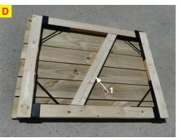
and lower 2x4 cross members (2x3" can also be basic frame. A cross brace is optional. (See #1) Turn used for cross members 2 x 4's must be used for side the gate over and insert screws through the fascia. members). Make sure to use 9 screws when attaching each bracket.
