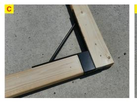
Attach the lower and upper brackets to the upper Fit the brackets together as shown. This will form the and lower 2x4 cross members (2x3" can also be basic frame. A cross brace is optional. (See #1) Turn used for cross members 2 x 4's must be used for side the gate over and insert screws through the fascia. members). Make sure to use 9 screws when attaching each bracket.
